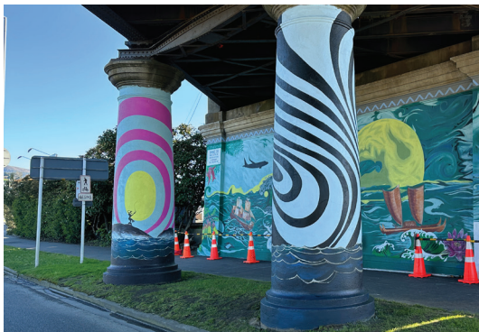
A new mural is brightening up Andersons Bay Road in South Dunedin.
