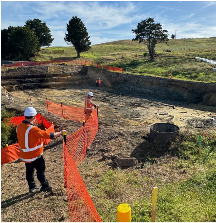
An example of Northland's slip prone geology. The excavation north of Waitira is where a gentle hillside slumped under the rail line. The track and ballast can be seen in the top left corner of the picture. This area will be rebuilt with sturdy material and improved drainage.
