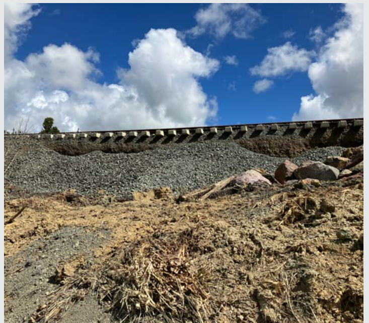
A major damage site near Topuni, which will be worked on over the Christmas break. Land under the rail line has collapsed and the entire 47 metre high slope will need to be retained, along with a new, larger culvert.
