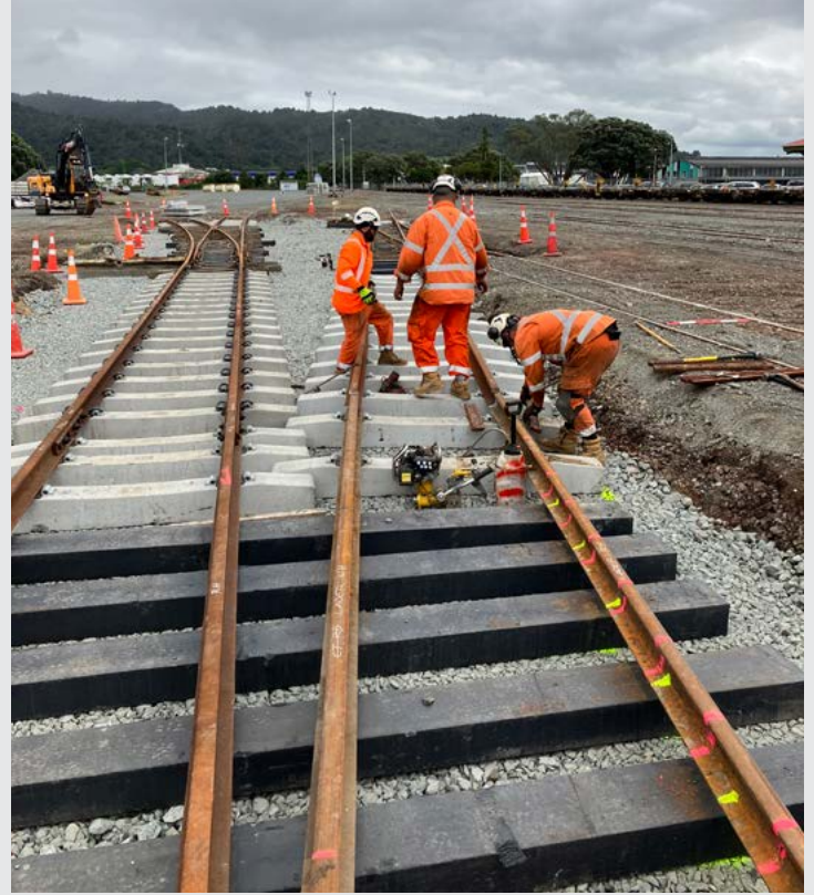
Upgrades to the Whangārei Rail Yard – old track foundations have been dug out and removed, geo-mesh put down and new rock laid. It is then compacted before the rails and track structures are reinstalled.
