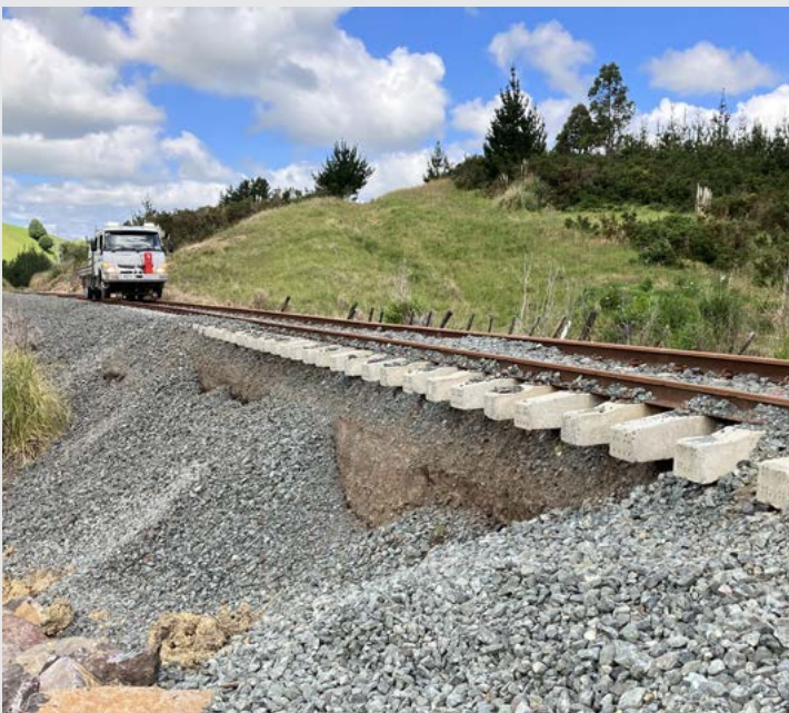
A major damage site near Topuni, which will be worked on over the Christmas break. Land under the rail line has collapsed and the entire 47 metre high slope will need to be retained, along with a new, larger culvert.
