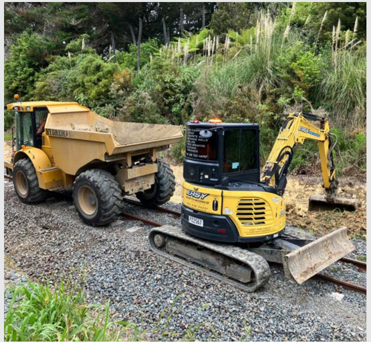
A swale drain being cleared near Maungaturoto.
