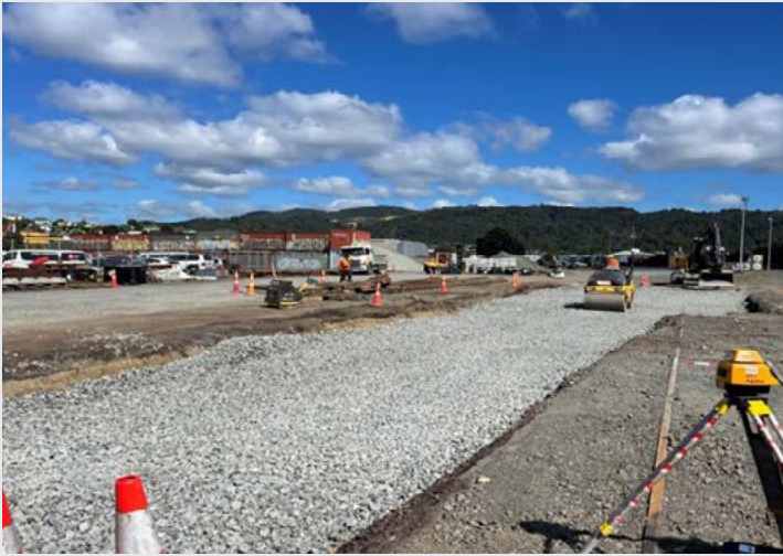
Upgrades to the Whangārei Rail Yard – old track foundations have been dug out and removed, geo-mesh put down and new rock laid. It is then compacted before the rails and track structures are reinstalled.
