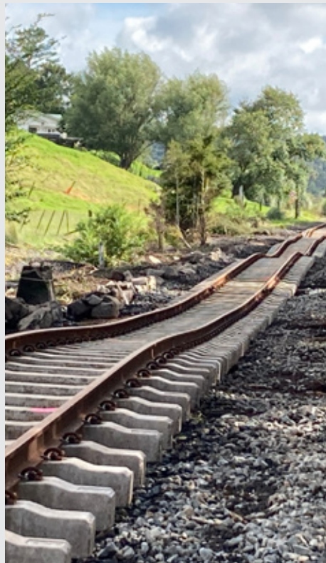
Rail damage near Kaukapakapa: track damaged after the 27 January flooding (left); repairs underway (top right); further damage in the 24 February weather event (bottom right).
