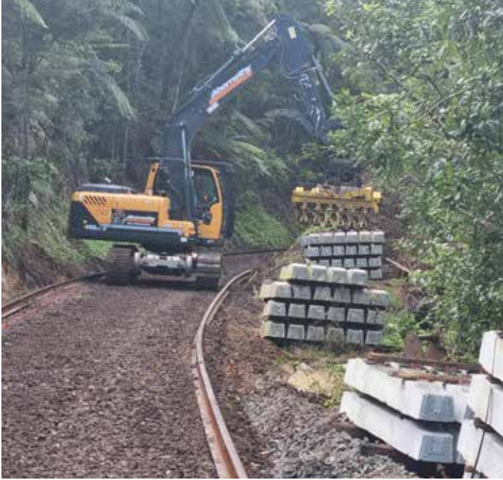
New rail and sleepers being installed between Waipanga Road and the Kauri siding
