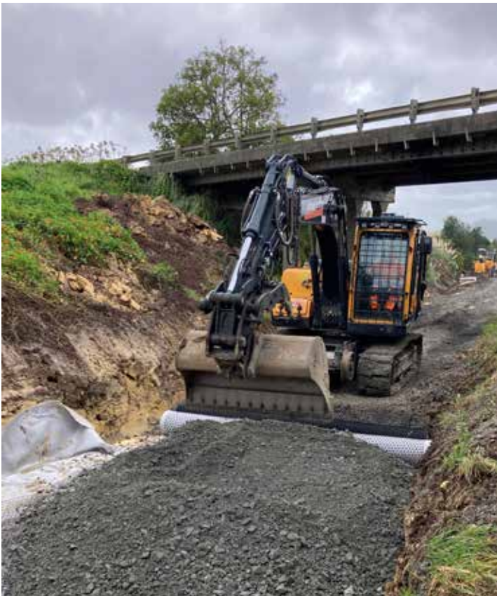
Rebuilding the track foundations and laying new sleepers near Kauri
