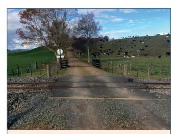
AN 'ASPHALT' LEVEL CROSSING consists of a base being prepared and asphalt laid over the level crossing to around 1.5 metres from the railway centre line. Asphalt level crossings require minimal maintenance and can last a long time before needing to be renewed depending on usage and topography of the land. Asphalt level crossings are also ideal for residential, lifestyle and some rural properties.
