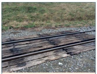
A 'TIMBER PANEL' LEVEL CROSSING consists of timber sleepers running parallel to the railway line. Timber panel level crossings require minimal maintenance and can last up to 20 years before needing to be reviewed. Timber panel level crossings are ideal for residential, lifestyle and rural properties.
