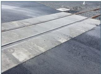
A 'CONCRETE (EDILON) SLAB' LEVEL CROSSING consists of concrete slab with inserted railway lines over the vehicle crossing. Concrete slab level crossings require minimal maintenance and can last a long time before needing to be reviewed. Concrete slab level crossings are ideal for level crossings with high vehicle usage, particularly by heavy-axle vehicles, and are suited to commercial and industrial type properties.
