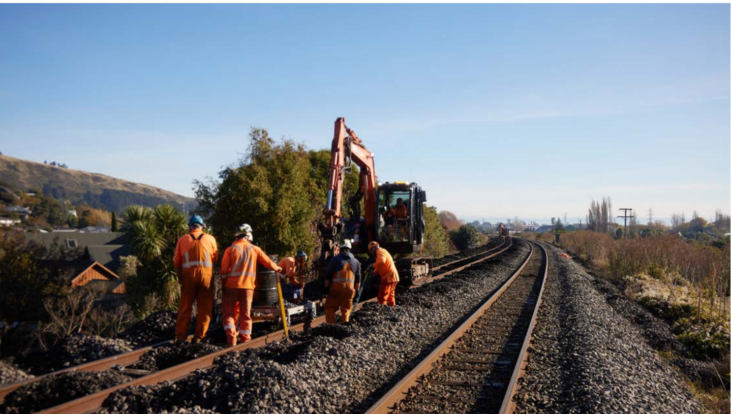
KiwiRail operates and maintains 3700km of track throughout New Zealand
