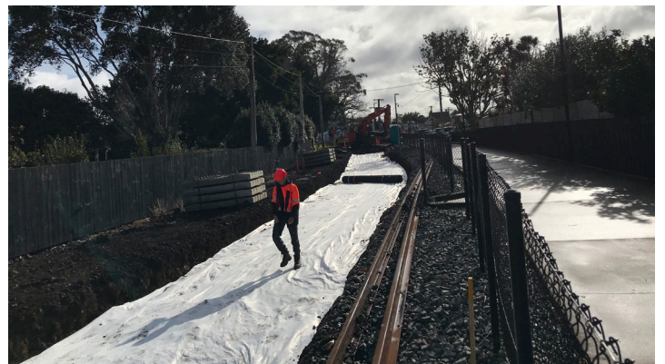
Preparing the formation bed between Manse Street and Vinery Lane in Whangārei
