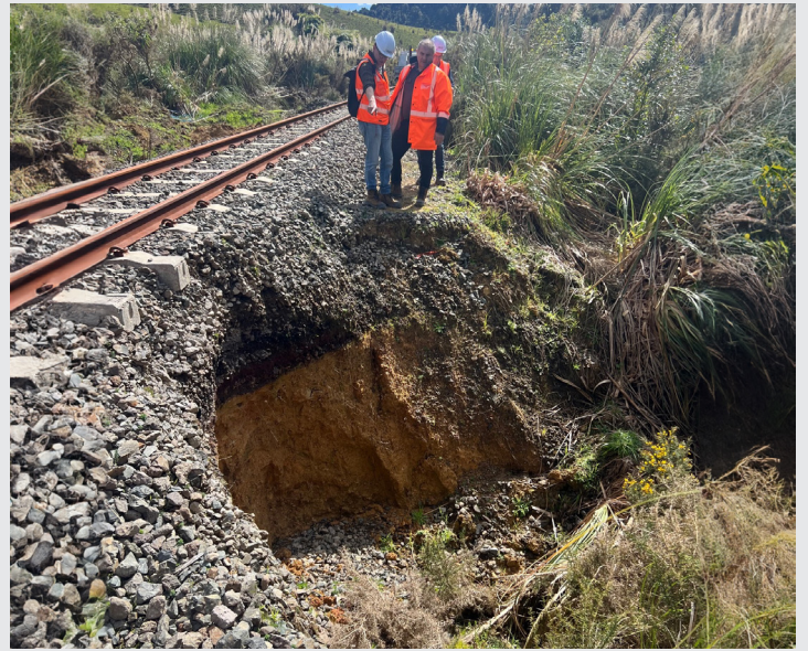
Examples of damage sites getting worse over winter: an overwhelmed culvert and a washout beneath the tracks, both south of the Kaipara Flats
