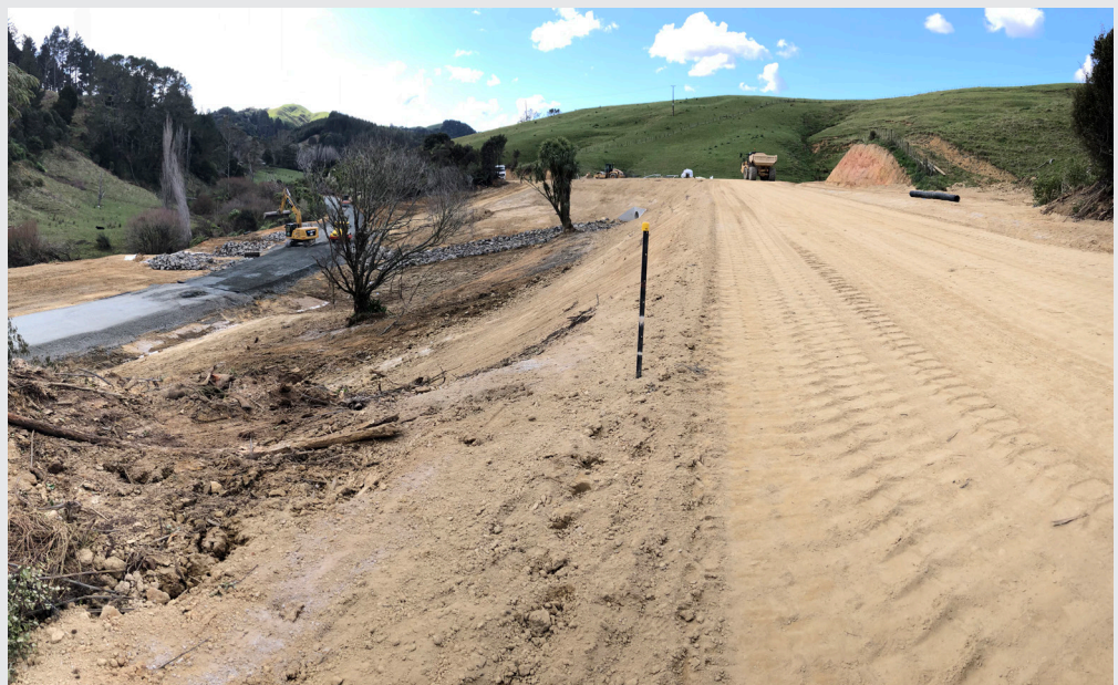
Tahekeroa - the 4m-high raised road just before surfacing began
