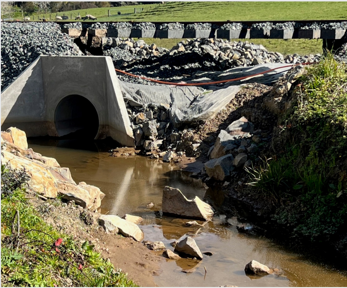
Examples of damage sites getting worse over winter: an overwhelmed culvert and a washout beneath the tracks, both south of the Kaipara Flats
