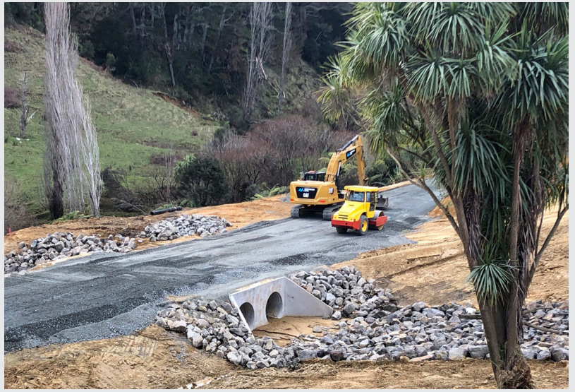
Takekeroa - rail formation being re-laid
