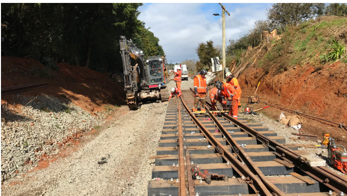
A turnout being built to connect to Fonterra's siding at Kauri
