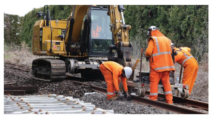
Timber sleepers being replaced with new higher strength and longer lasting concrete sleepers.
