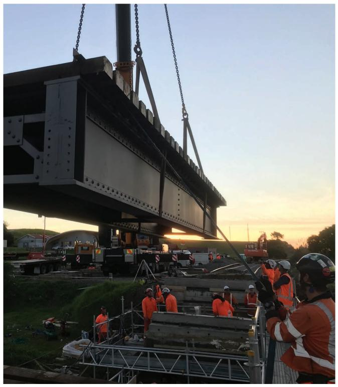
Refurbished steel span being lowered into place.
